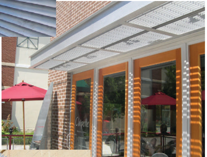
VisiShield panels placed horizontally provide solar protection at building entrance.
